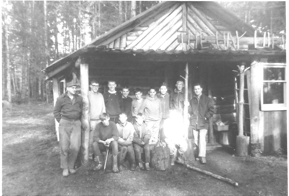
One of the 15 log buildings built at Camp Couch on Camano Island by one of the Scout Groups. Photograph 94.75 Courtesy Viola Couch.
