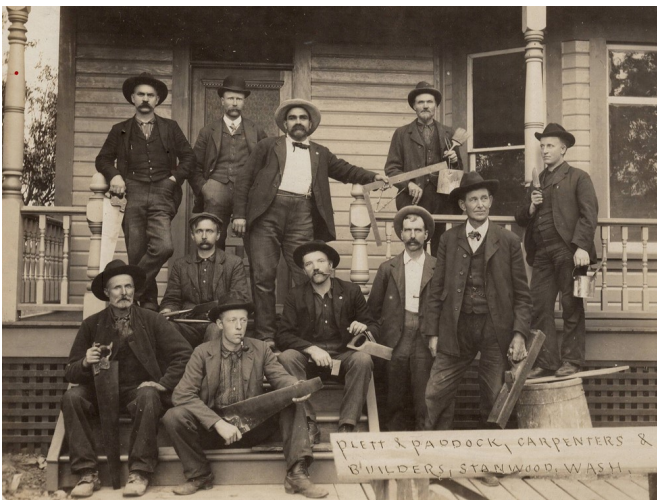
Plett and Paddock, Carpenters & Builders, Stanwood, Wash. SAHS Acc# 88.06.139.12
