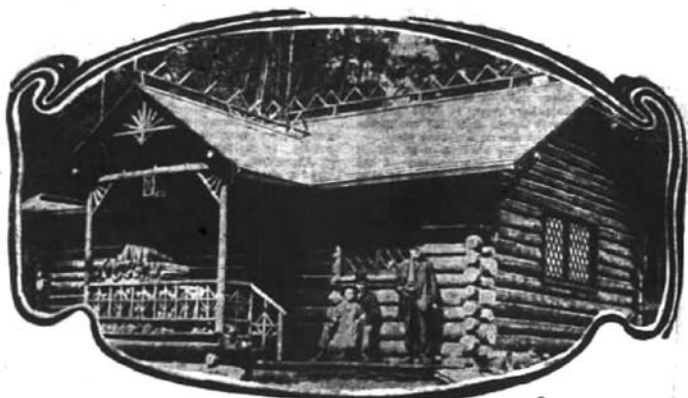
Mr. and Mrs. Charles Eugene Banks Cabin in Process of Construction Waupello Colony, Camano Island, Puget Sound.
